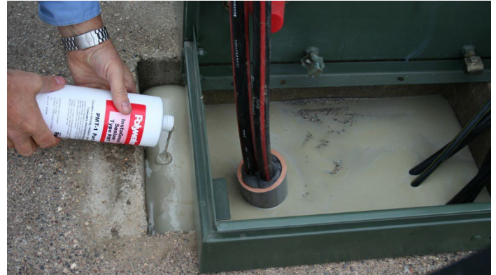
InstaGrout repairs and creates a barrier for cabinet bases.
